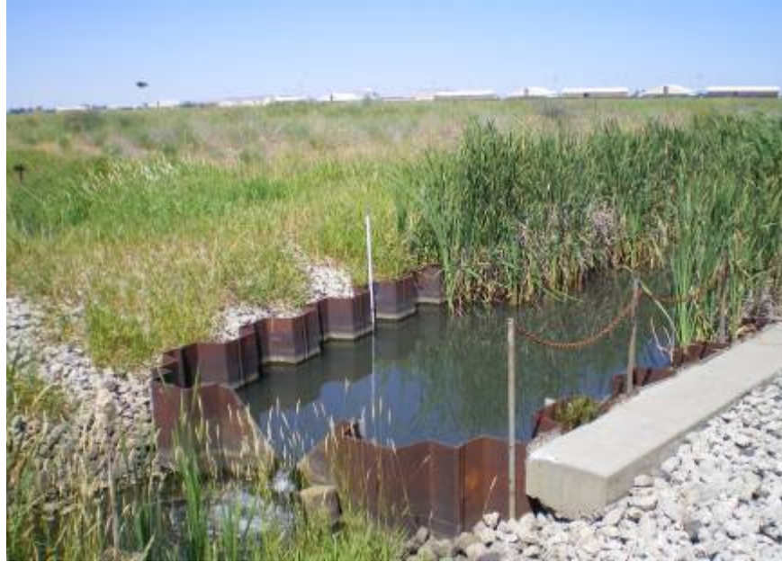
FIGURE H-1 DRAINAGE BASIN 1 OUTFALL
