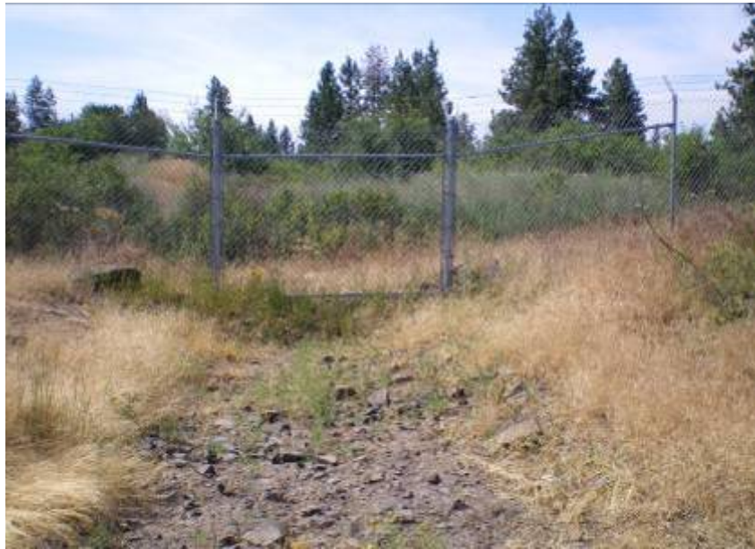
FIGURE H-4 DRAINAGE BASIN 7 OUTFALL
