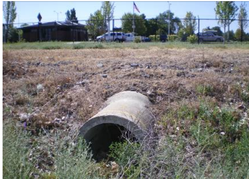
FIGURE H-2 DRAINAGE BASIN 3 OUTFALL
