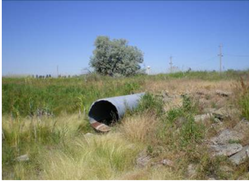
FIGURE H-3 DRAINAGE BASIN 6 OUTFALL
